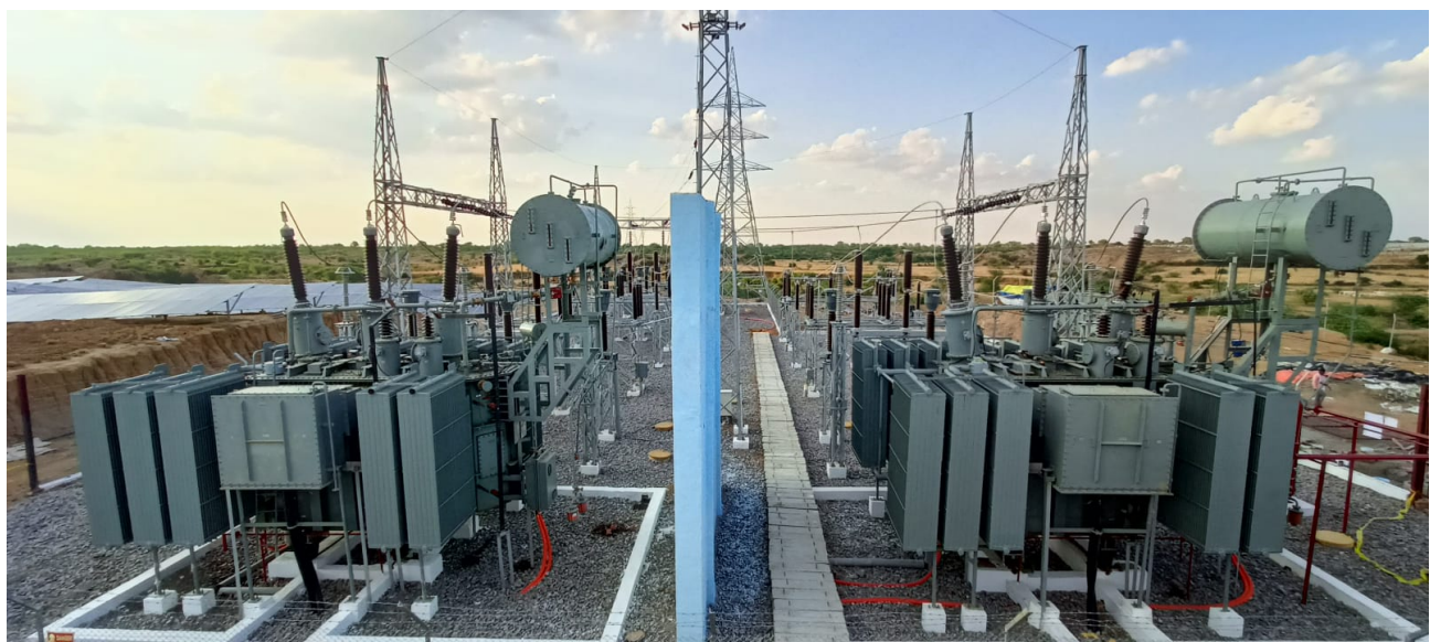
33 MVA Power Transformer- 2Nos
