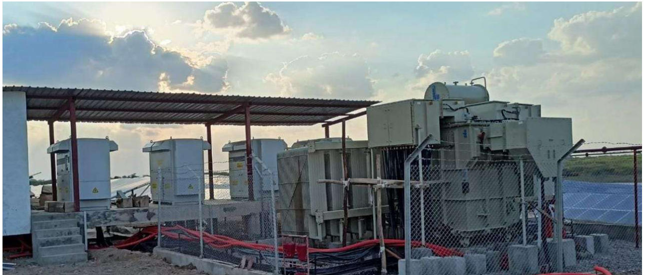
Block-1 Inverters with 13MVA Inverter Duty Transformer
