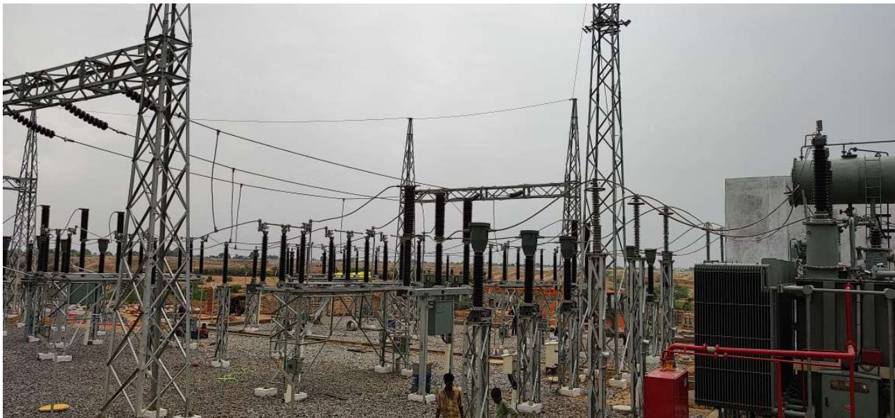
132kV Switchyard-Pooling Sub-Station
